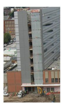
In the first week of August, the subcontractor, Eastern, will be re-mobilized to erect the final panels on the east side of the bed tower. Upon completion, the exterior skin will be 99 percent enclosed with exception of the cladding panels by the connecting bridge (which should be completed in September) and then a couple of leave outs for delivery purposes.
